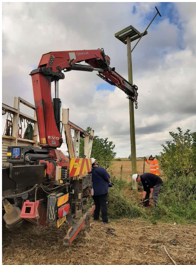
The new nest platform being installed at Site K with the assistance of National Grid © Tim Mackrill
